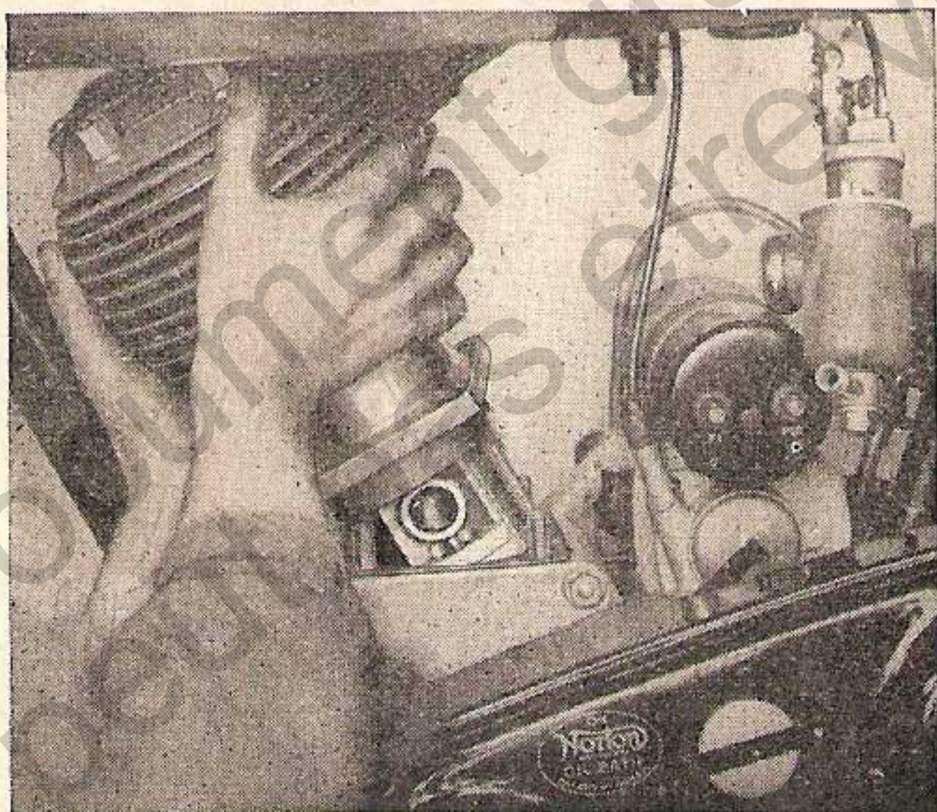
Removal of Cylinder Barrel.
