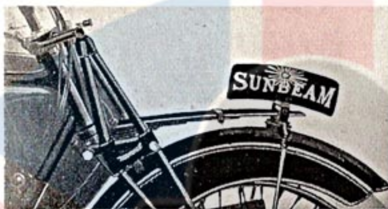
LEAF-SPRING FRONT FORK ON MODEL 7
