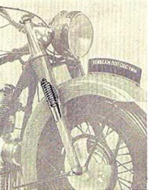
Superb steering is provided by the telescopic front forks fitted with automatic progressive hydraulic damping.
